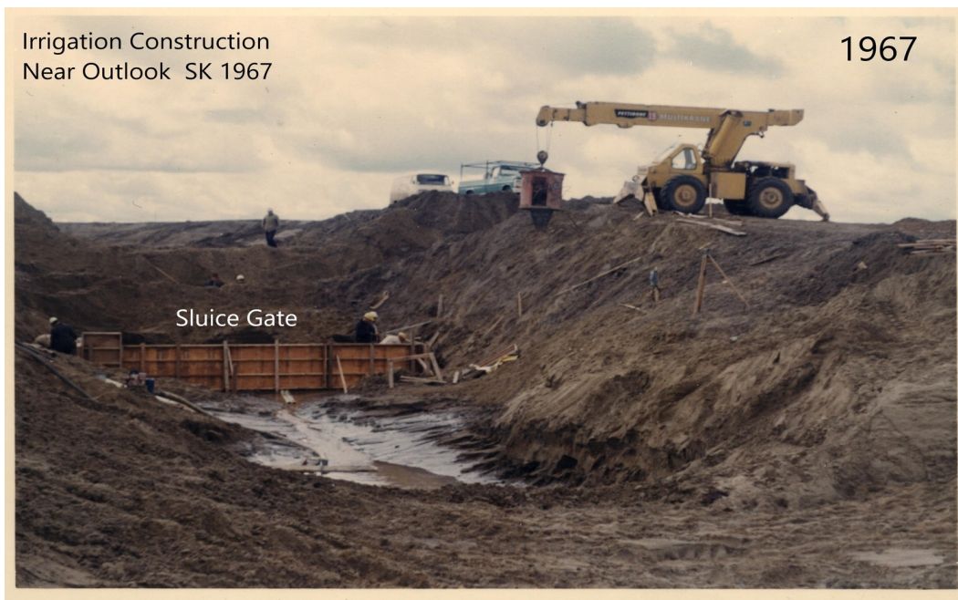
Photo 58 Constructing Water Supply Canal and Control Structure (1967)
